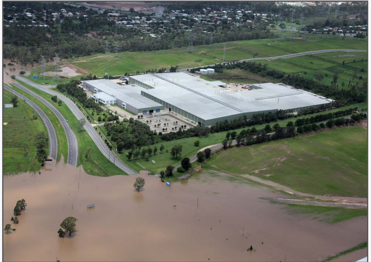
January 2011 floods Capral Bremer Plant Ipswich QLD
