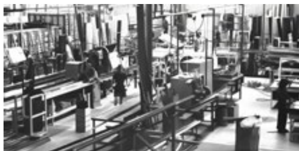
Residential window & door area, 1977
