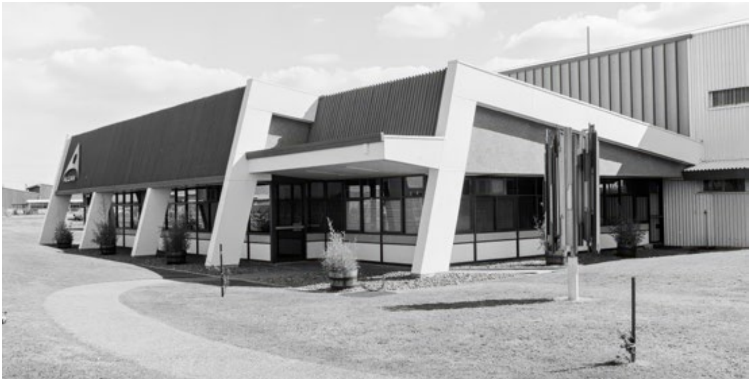
Eagle Farm admin building, 1972
