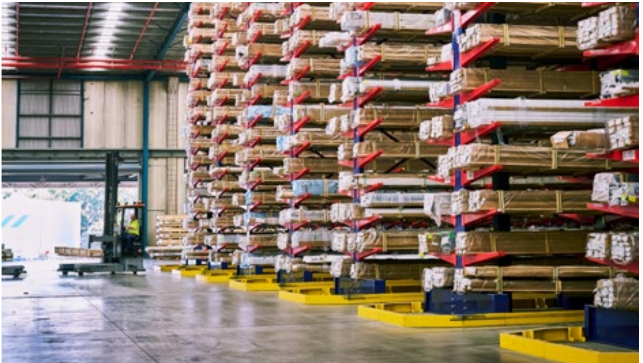
Huntingwood RDC warehouse, NSW
