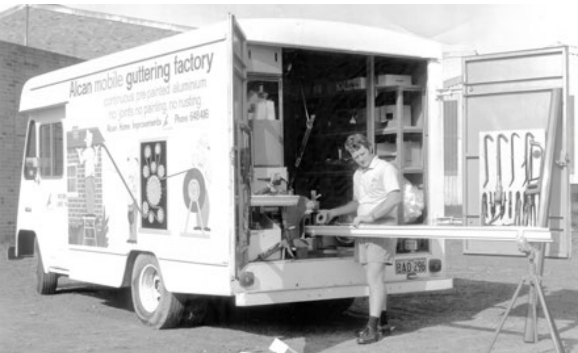
Alcan's mobile guttering service brought aluminium gutter forming and installation directly to building sites, 1970s.
