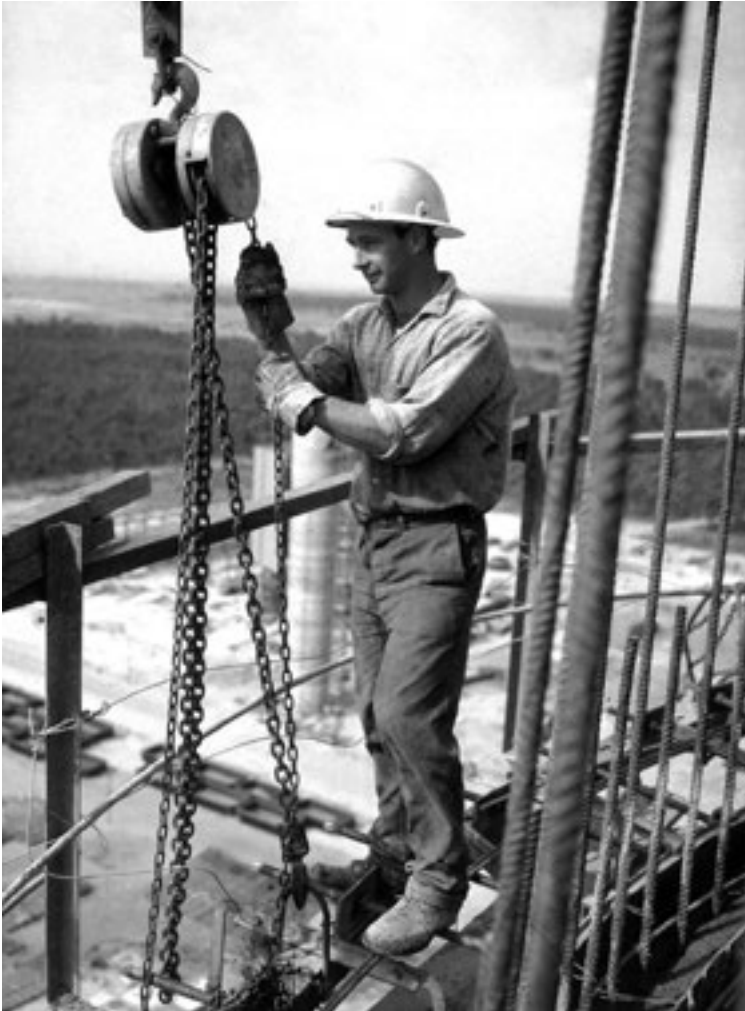
Construction worker at Alcan Kurri Kurri, 1968. Photo by Greg Ray.
